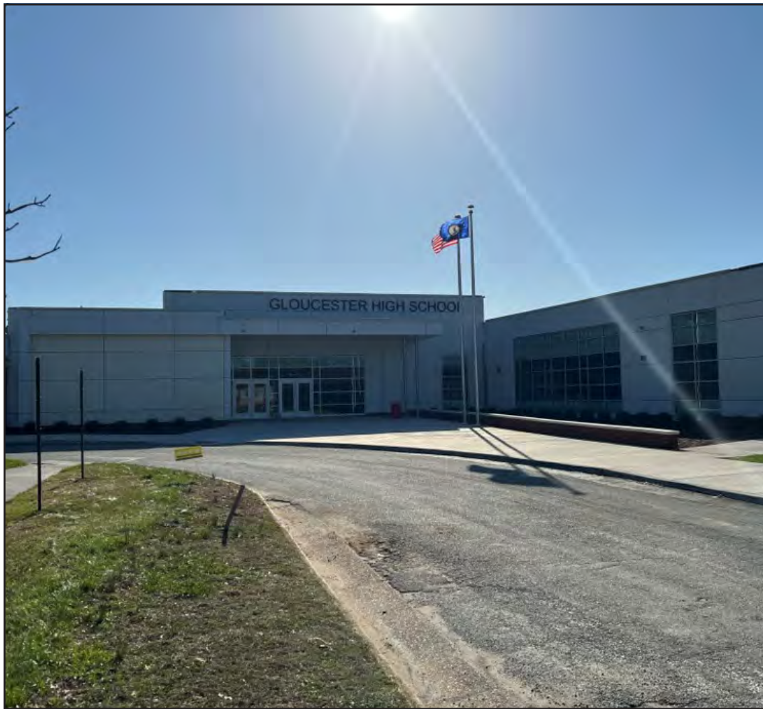
The Gloucester High School renovation project has a busy summer planned. Pictured is the new front entrance, which was completed earlier this school year.
