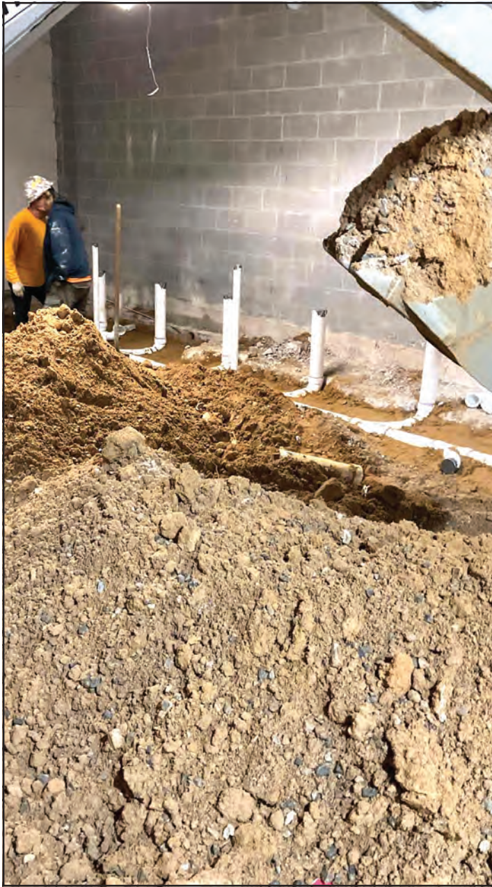
Construction of new inclusive restrooms.
